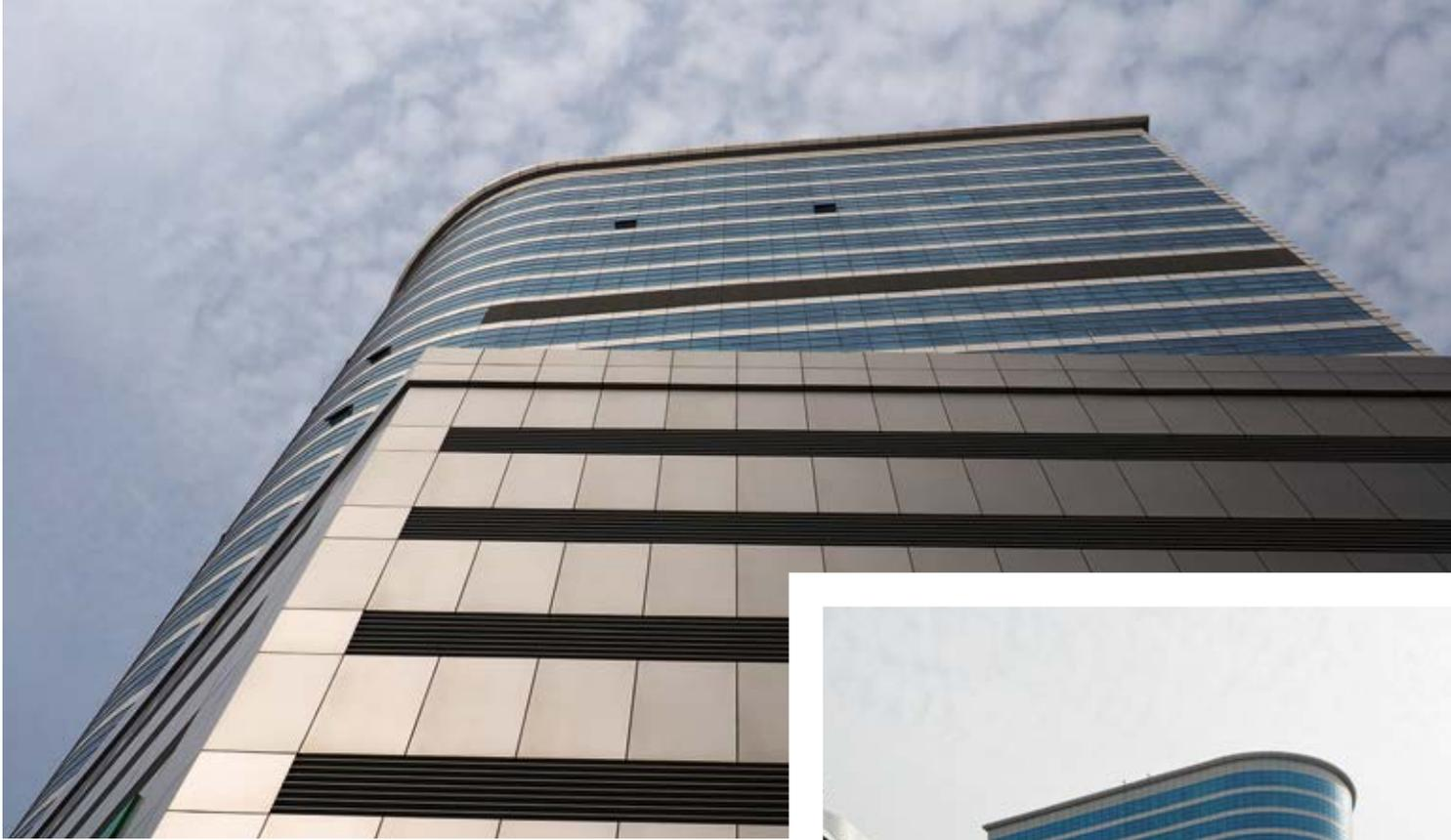
The HUECK Lambda 110 system rounds off this ambitious façade with highly thermally insulated aluminium windows, to which the planners devoted their particular attention in this climate zone with its high temperatures. ➔
